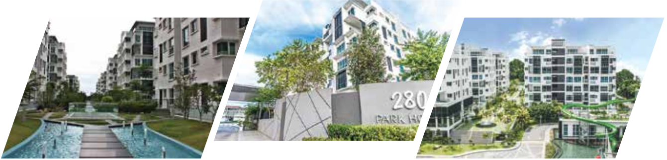
280 Park Homes, Puchong (Malaysia)
